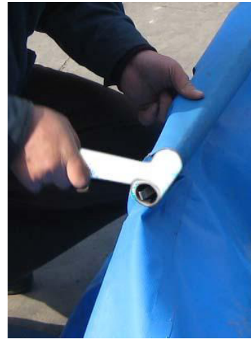
Step 12: Attach the short connector tube to the long connector tube
