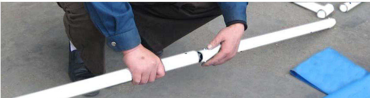
Step 12: Attach the short connector tube to the long connector tube
