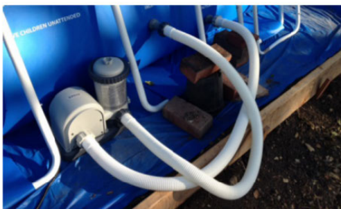
Filter Pump Connection
