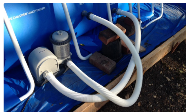
Filter Pump Connection
